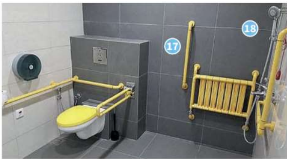
Figure 5: Examples of orientation cues for quick identification of the toilet. Good contrast of colours for fixtures and fittings.
