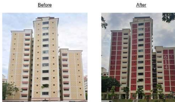
Photo 6: Colour zoning, enlarged block numbers and contrasting colored vertical strips to the public housing estates to help better wayfinding within the neighbourhood.
